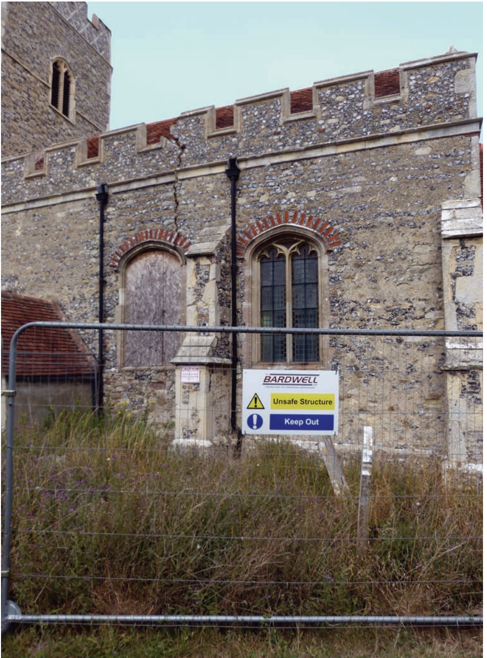
Major repairs including underpinning at Althorne, St Andrew. © James Bettley
