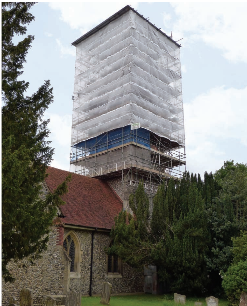
Spire repairs at Manuden, St Mary the Virgin. © James Bettley
