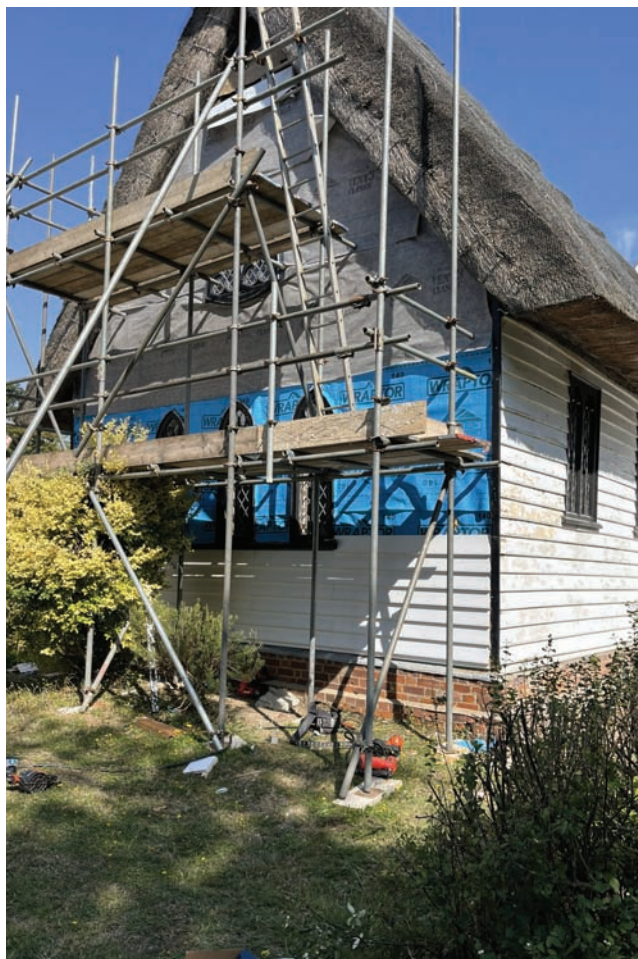
Roofing and other repairs at The Hamlet Church, Duddenhoe End.
