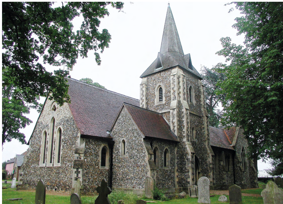
Guttering and associated repairs at Hatfield Heath, Holy Trinity. © James Bettley
