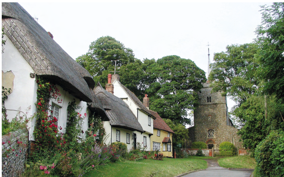
Roof repairs to chancel at Wendens Ambo, St Mary the Virgin. © James Bettley
