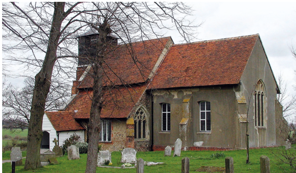
Window masonry repairs at Buttsbury, St Mary. © James Bettley
