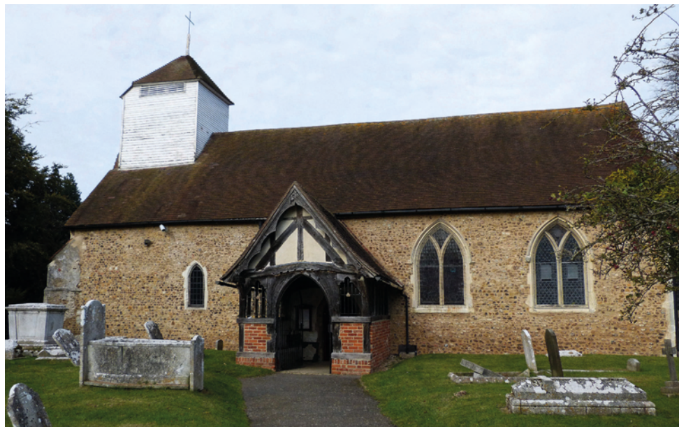
Roof repairs at Little Clacton, St James. © James Bettley
