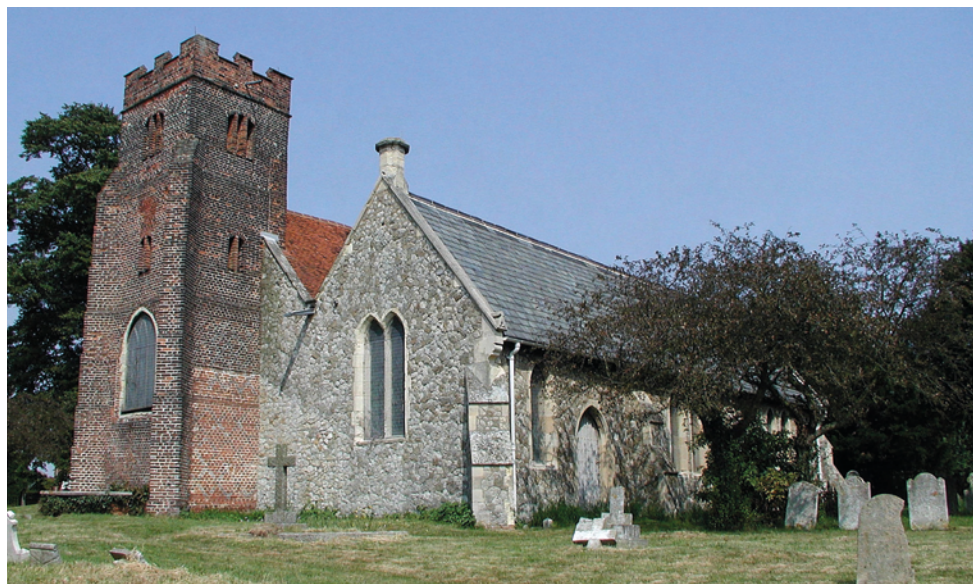
Retiling of nave roof at Greenstead (Colchester), St Andrew. © James Bettley
