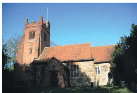
Gutter and rainwater pipe repairs for Inworth, All Saints
