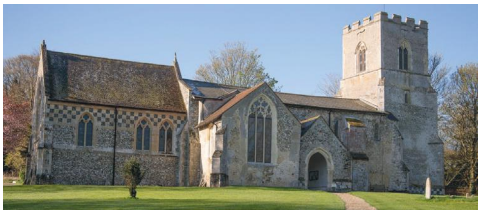
Repairs and a nave roof walkway for Hadstock, St Botolph
