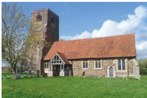
Ceiling plaster repairs for Tolleshunt Major, St Nicholas
