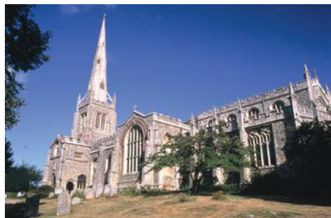
Window repairs for Thaxted, St John the Baptist
