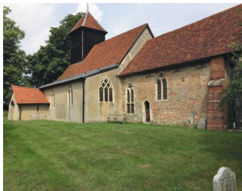
Level floors and improved access for Alphamstone, St Barnabas
