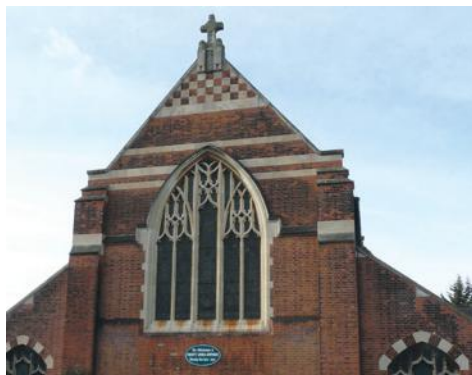
Window repairs for Goodmayes, St Paul
