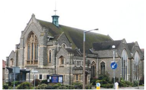
Roof repairs at Westcliff Crowstone © L Denton
