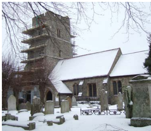
Paglesham: work in progress, December 2010
